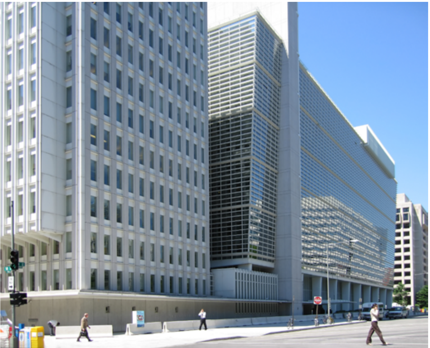
World Bank building, Washington, DC. Photo by Shiny Things on Flickr .
